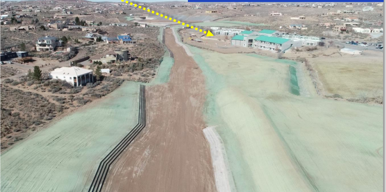
Photo# 2 - Lomas Negras Post-Construction 2020
