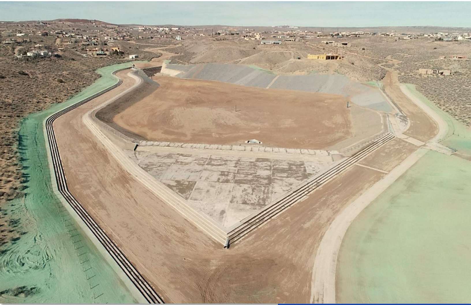
Lomitas Negras Post-Construction 2020
